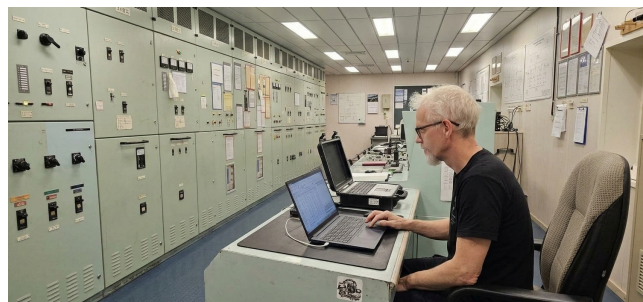
Reading measurement data in the engine control room.
